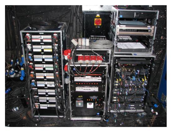
Mains distribution equipment backstage. The rack on the left is a 108 x 10 Amp channels of single phase power distribution, in the centre is a 16 way three-phase distribution unit, the rack on the right is control data distribution.
