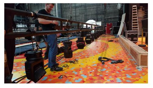
Lighting being rigged and cabled onto a theatre's fly bar at stage level, before it is flown out to a show height of around eight or nine metres.
